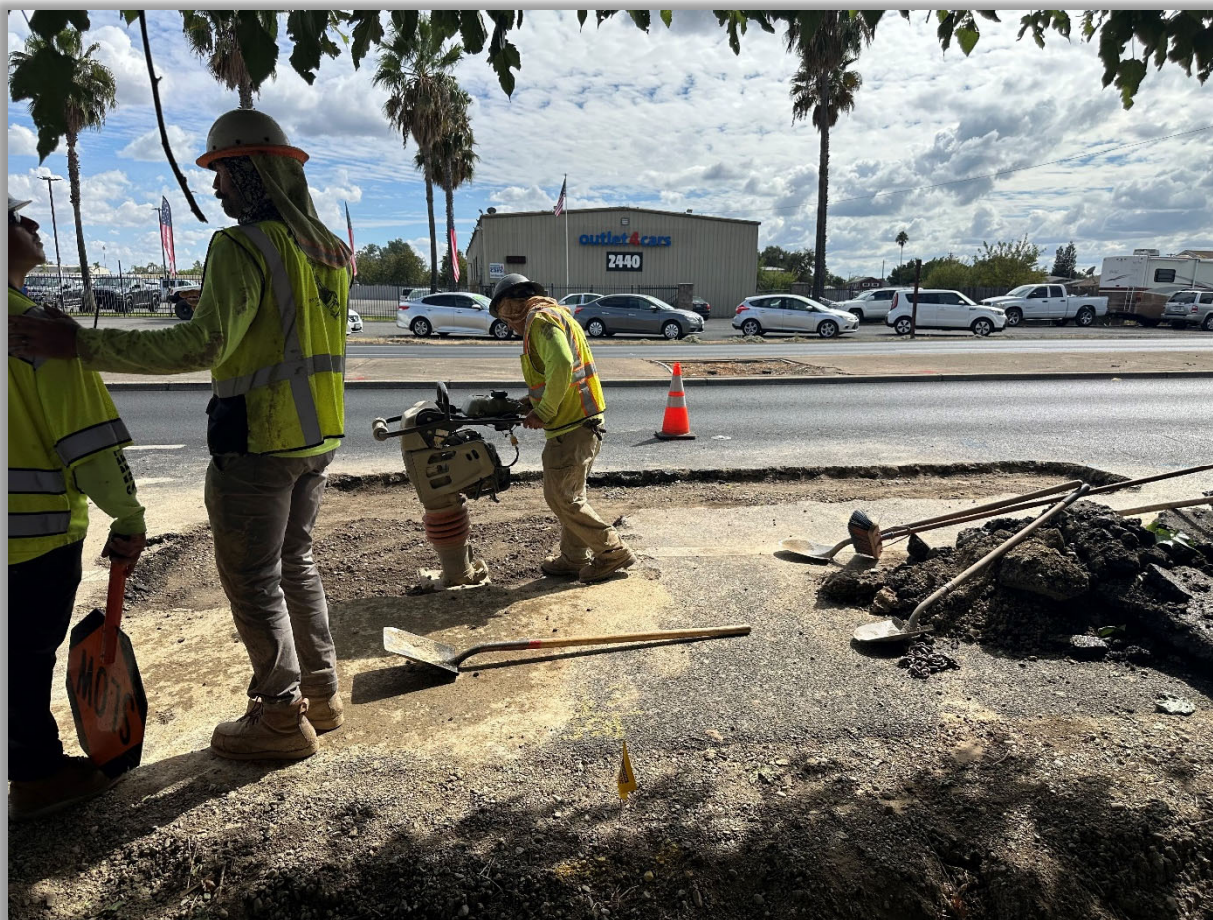
Leak Repair North Side of Elkhorn Blvd. between 24 th and 26 th Streets
